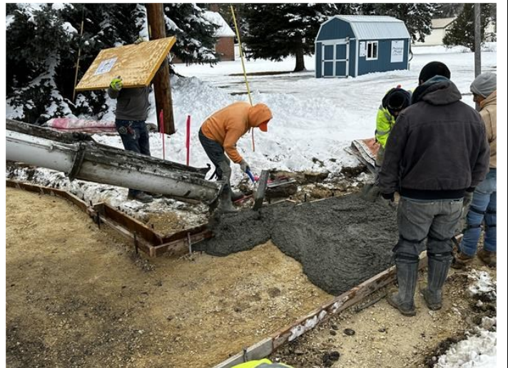
Subject: Concrete placement via truck and chute
