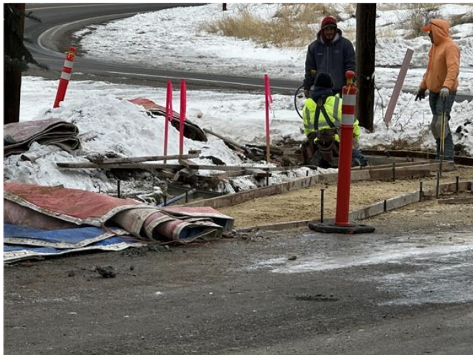
Location: Vaughn Street corner looking Southeast
