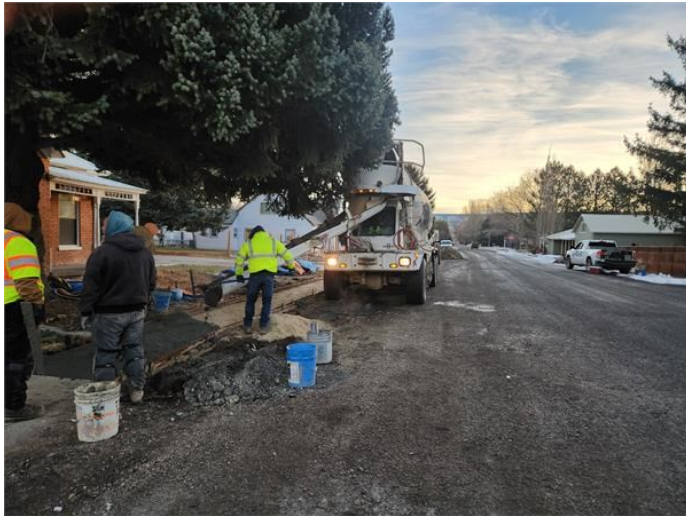
Location: W Market Street Concrete placement looking East.
