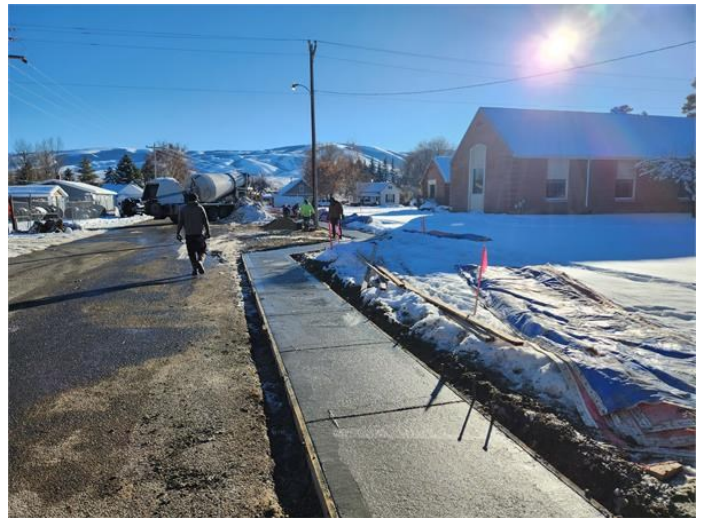
Subject: Concrete placement via truck and chute.
